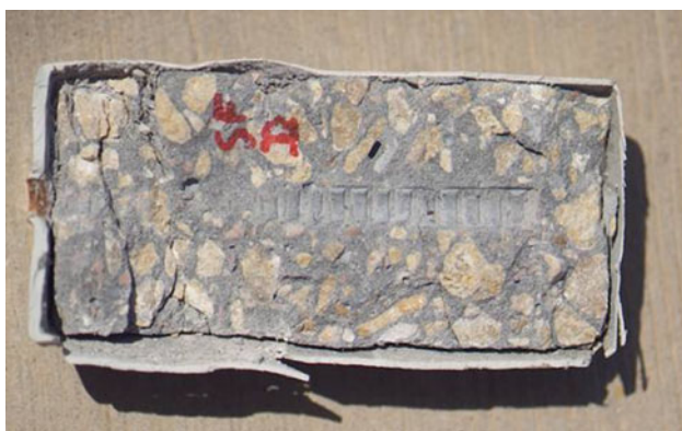
Fig. 15 Photograph showing detachment of the coating from the concrete substrate
